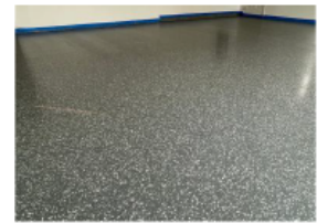
Epoxy Flake Flooring
